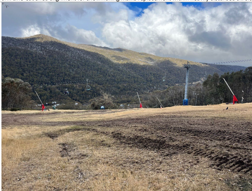
Cat Shed-Milk Run split alignment for snowmaking mains and laterals replacement. Trenching within heavily disturbed ski slope.
