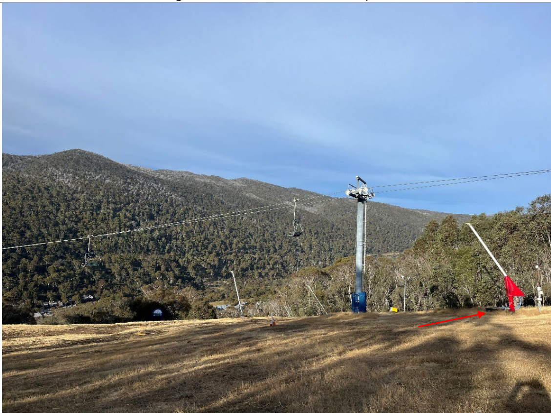
Existing pit and lance gun to be replaced with new fan pit, TT10 fan gun and lateral from snowmaking mains.
