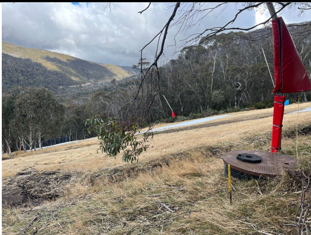
Tree island at top of Milk Run ski run. Fan pit and TT10 fan gun to be installed next to existing pit and lance gun. Lateral connection to new snowmaking mains line downslope.
