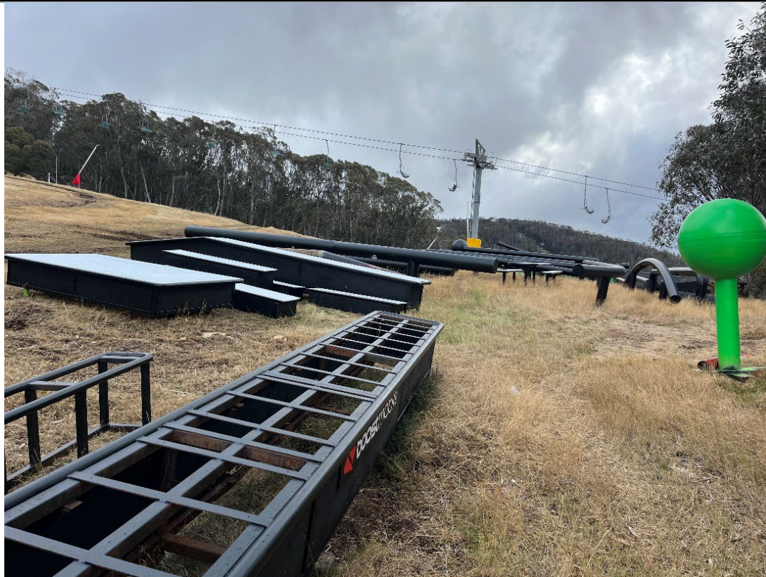
Trunk Line -Cat Shed alignment for snowmaking mains replacement. Trenching within heavily disturbed area dominated by exotic grass species.
